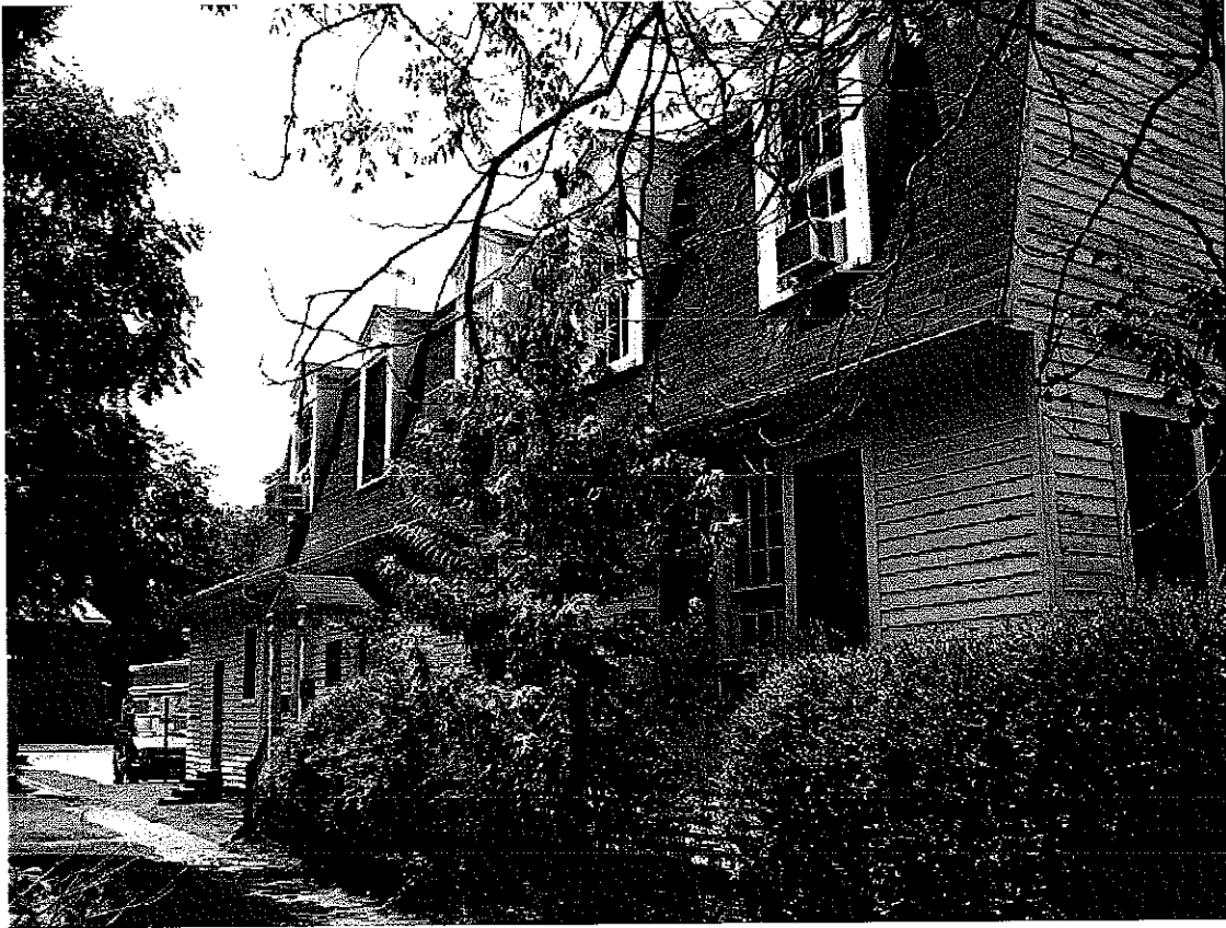
Figure 12. Northeast corner of Prince George Street House, 2005.
