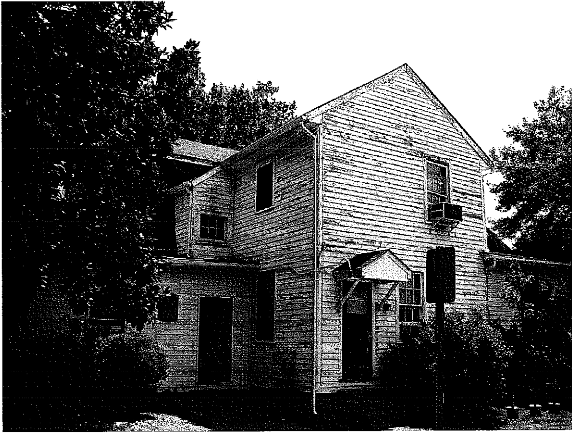
Figure 13. Northwest corner of the Prince George Street House.
