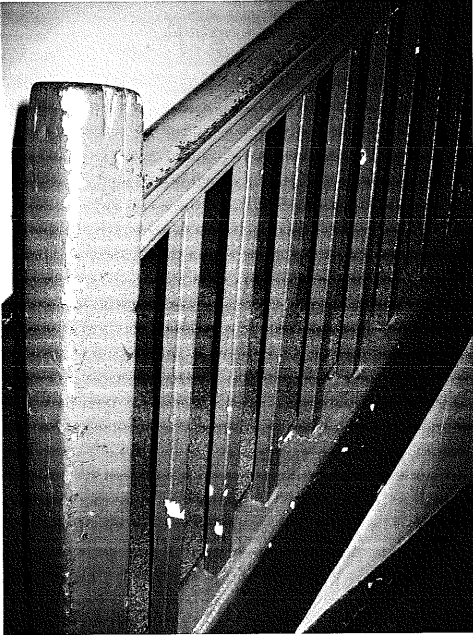
Figure 15. Detail of newel post, lower balusters and handrail of early stairs.
