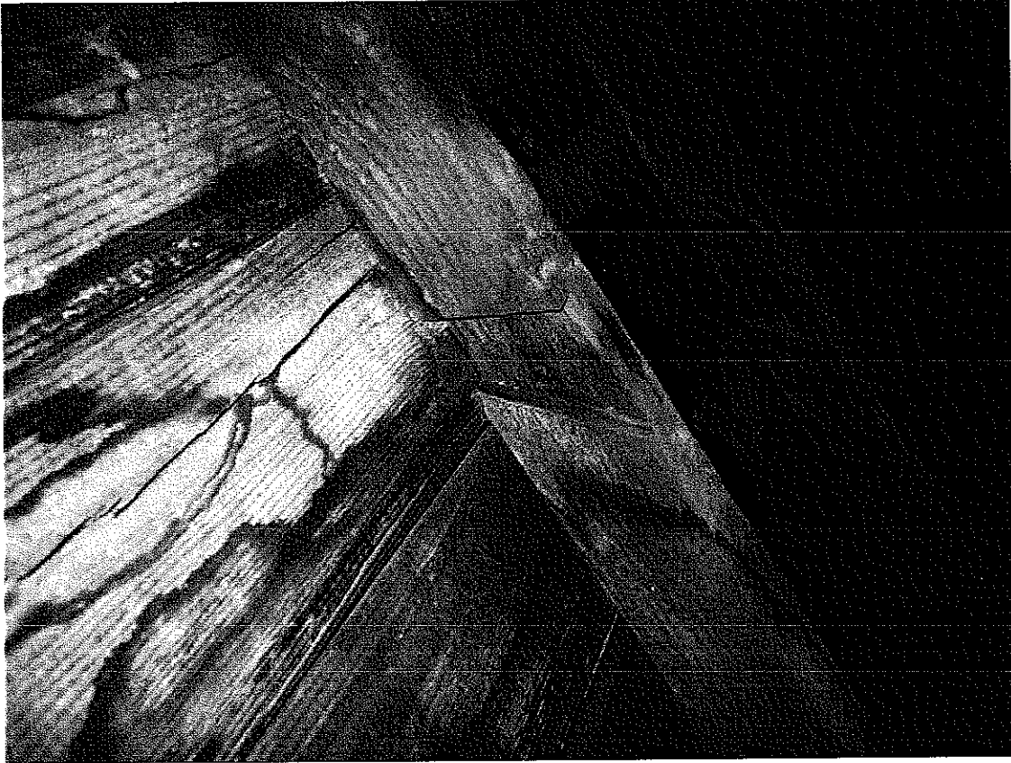
Figure 17. Reworked Period I rafter with empty dovetail joint and a wrought nail.
