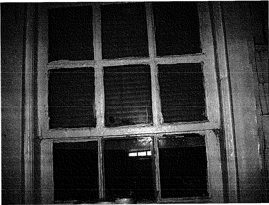
Figure 14. Exterior view of Period I upper sash on parlor window.
