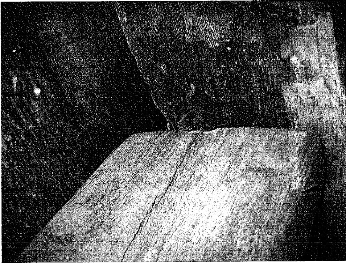
Figure 20. Pegged joint in framing below Period I structure.
