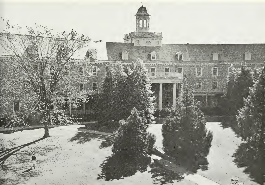
Barrett Hall from the Campus side
