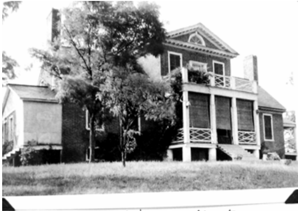
Photo 1930's before the disastrous alterations (view from southeast)
