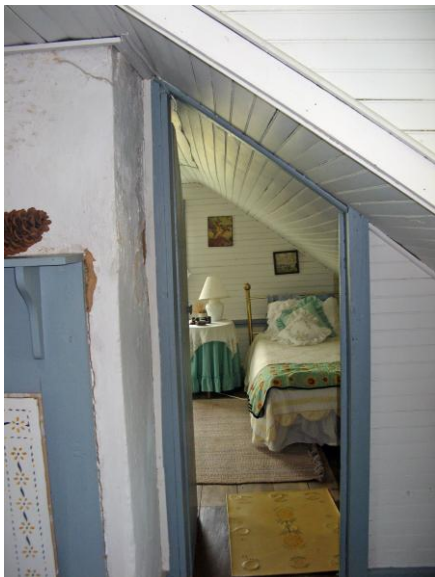
Passage Leading Between 2 Upstairs Bedrooms
