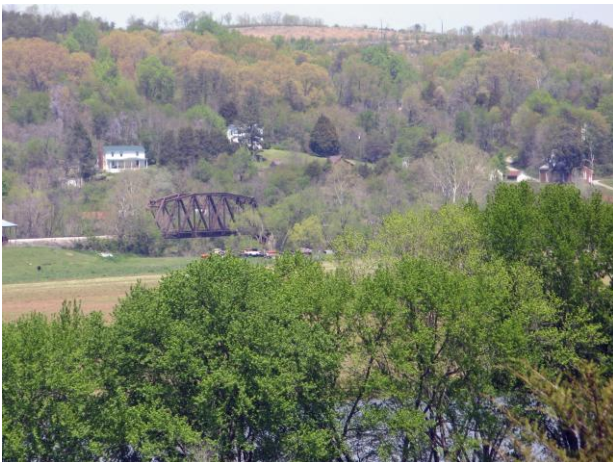
View of Bridge over Tye River from Green Hill
