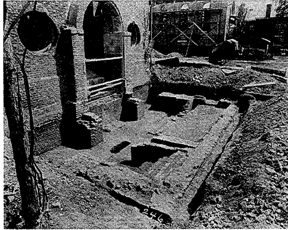
Fig. 16. Foundations of the Hall of the First College Building, 1929, photograph: Colonial Williamsburg Foundation.
