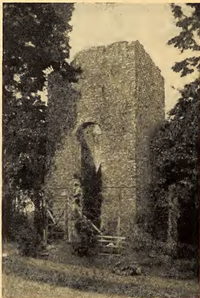
OLD CHURCH TOWER
