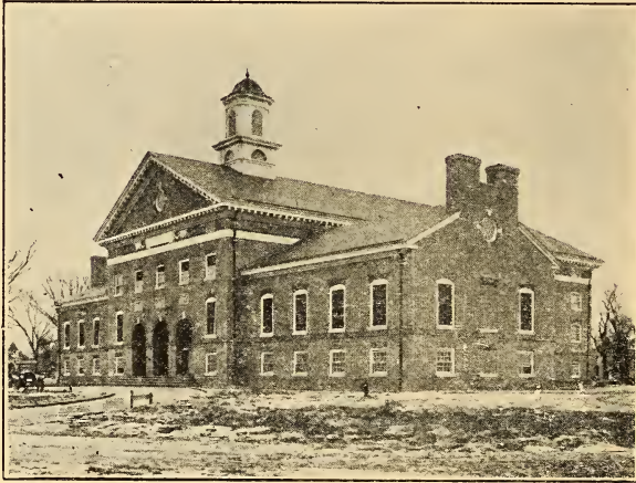
George Preston Blow Gymnasium
