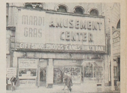
OLD FRONT will come down shortly with new fixtures on order to brighten the appearance.
