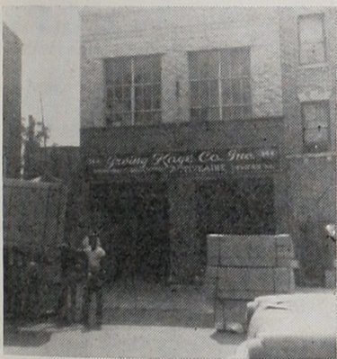
Loading dock is at far end of block long plant.
