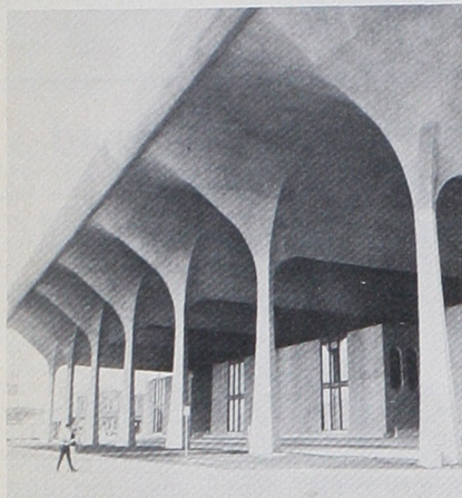
Entrance to the Rivergate Exhibition Hall
