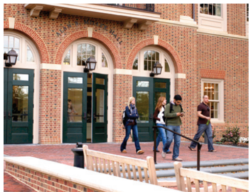
SUN PARK — THE FLAT HAT Currently, the newly constructed Miller Hall closes at 10 p.m. to students not taking a business class.
