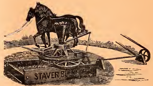
STAVER BUCKEYE COMBINED MILL AND POWER.
