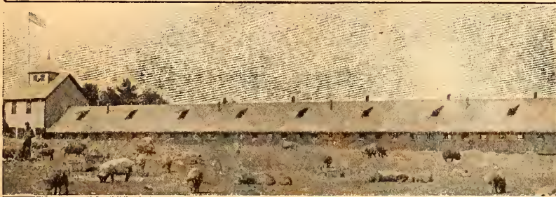
ONE OF THE BELLEMEADE FARM BUILDINGS ROOFED WITH AMATITE.
