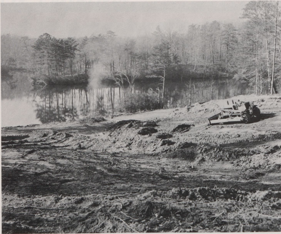
Early stages of construction of theatre, 1947.
