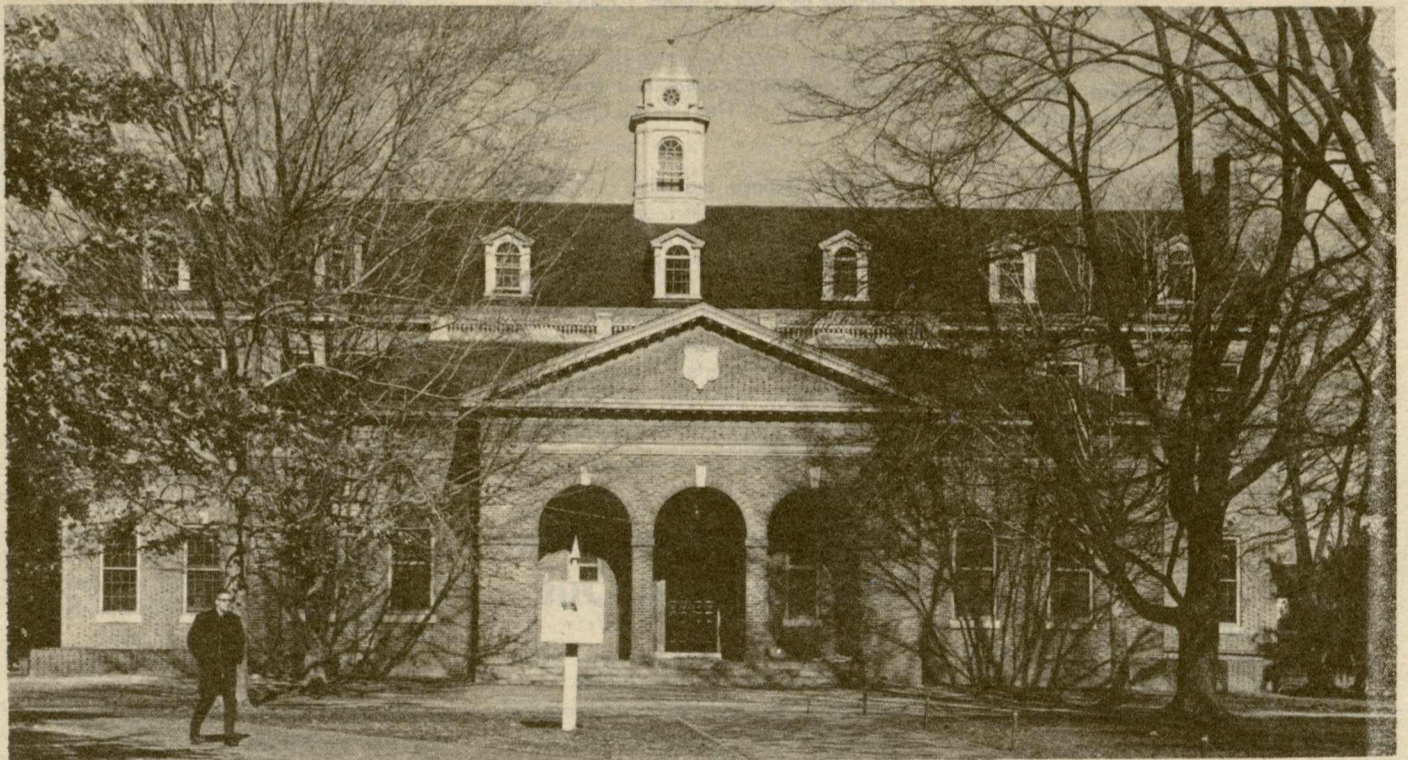
The Marshall-Wythe School of Law building, soon to be vacated in favor of new quarters adjacent to the National Center for State Courts, will get a new name when its present tenants leave. Marshall-Wythe will become St. George Tucker Hall when the law school moves to its new quarters.
