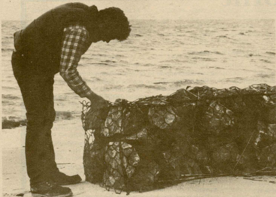
VIMS erosion specialist Scott Hardaway inspects a gabion.
