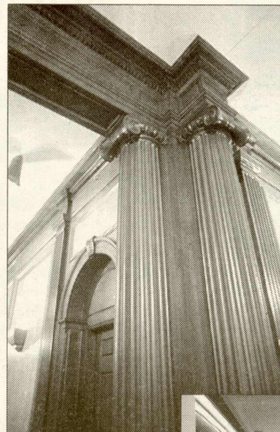
Where old meets new: Blair's stately walnut paneling was carefully preserved during the renovation, while state-of-the-art instructional technology was installed in many of the building's classrooms.
