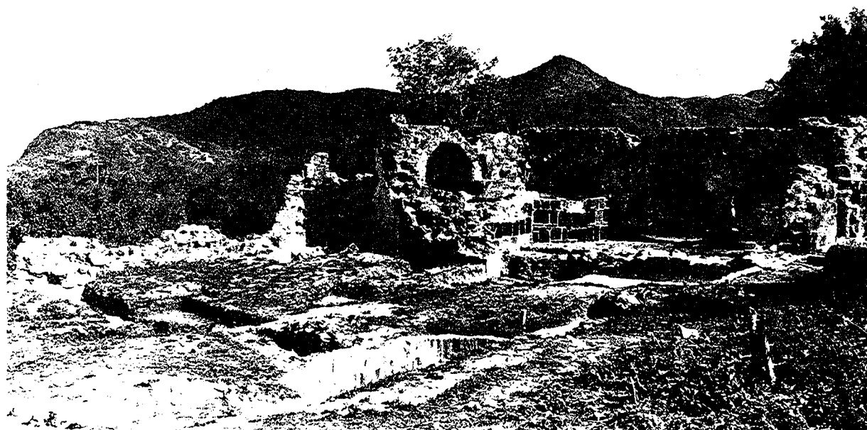
Figure 4. The north end of the building, looking south.
