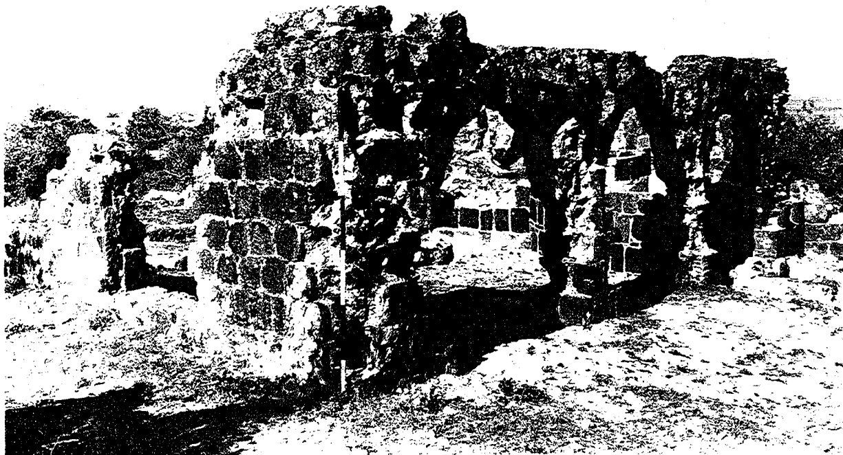
Figure 21. Northeast corner of building (Room 2), looking southwest.
