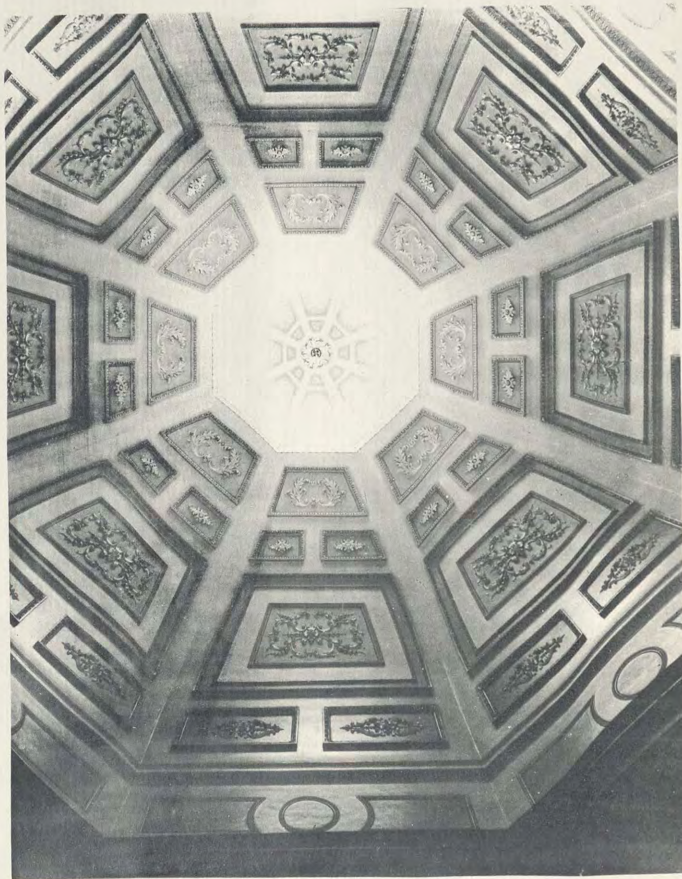
PLASTER WORK AND LANTERN IN DOME OF ANTE-CHAPEL AT CLARE HALL, CAMBRIDGE UNIVERSITY
