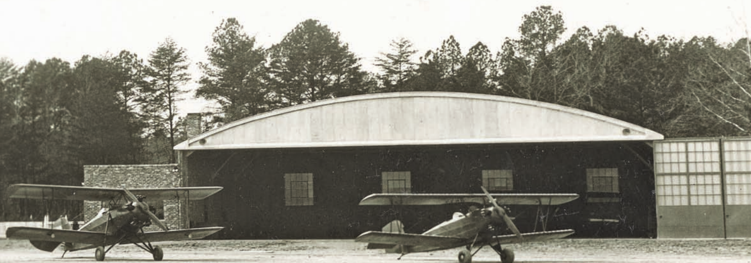
Field equipment of William and Mary Air School: Curtis Robin, two Kitty Hawks and one Fleet. The $10,000 hangar was equipped with waiting rooms, offices and shops. Photo courtesy of Will Molineux '56.
