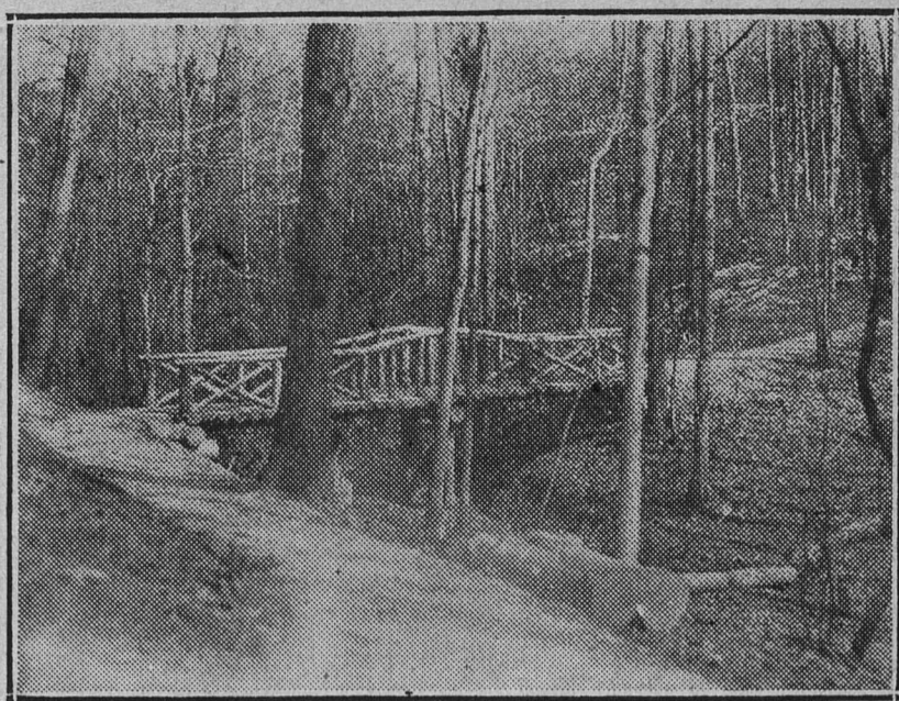
Squirrel Hollow Bridge in Matoaka Park.
