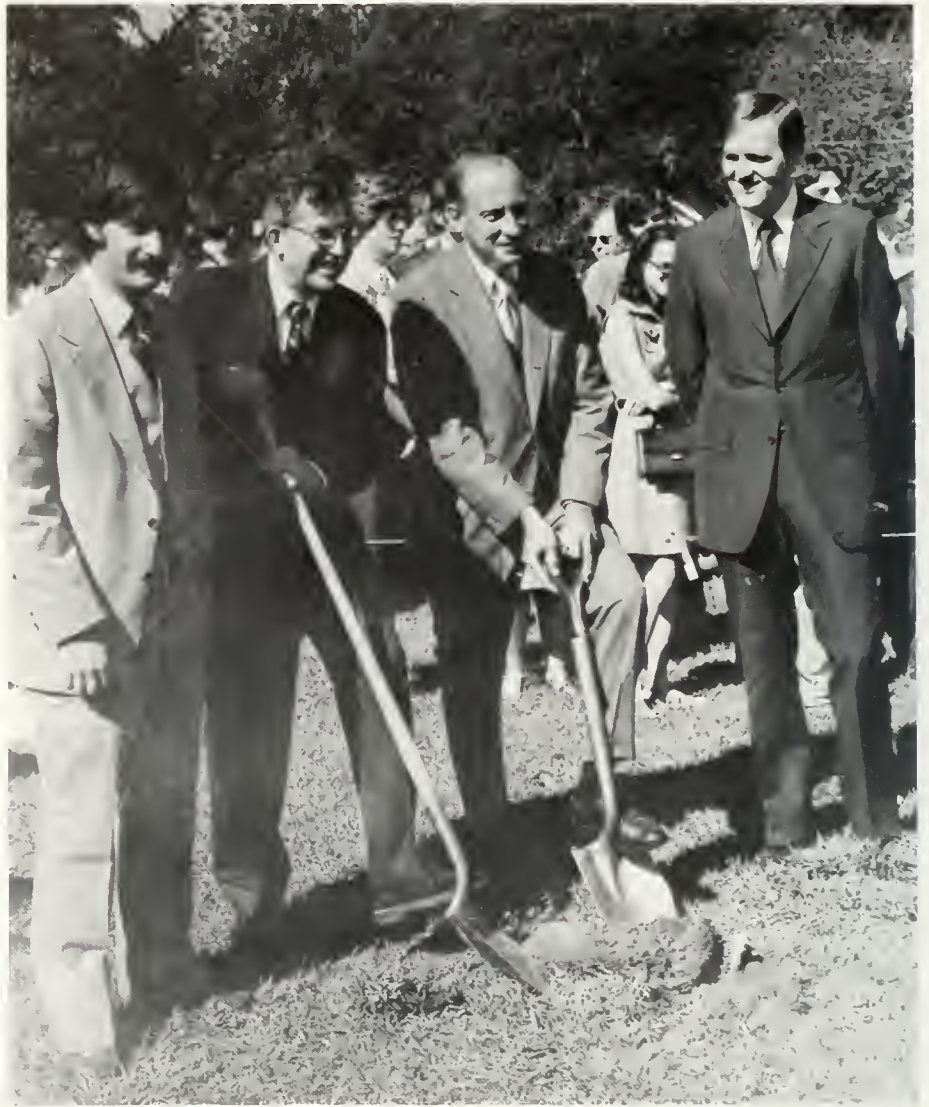
A spade in hand. President Graves breaks ground for the new Law School.
