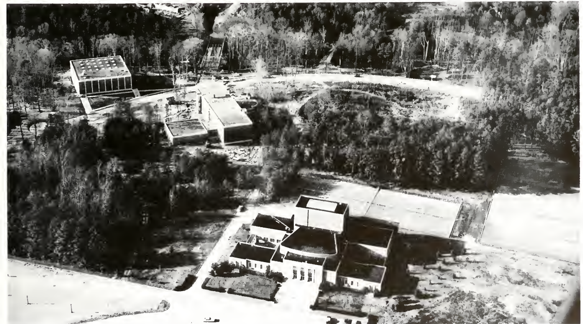
Aerial view of new campus.
