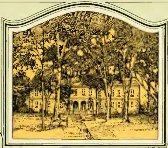
Main Building Today
