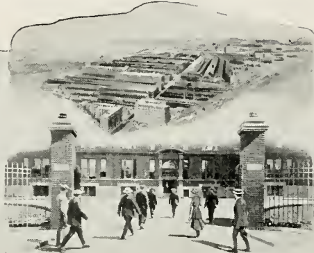
MAIN PLANT GENERAL ELECTRIC COMPANY
