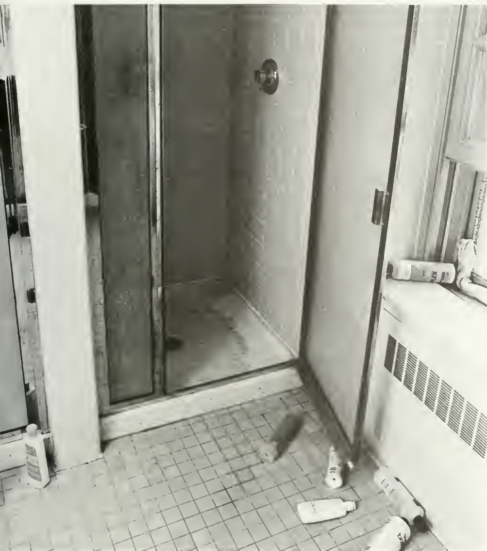
◀ Jefferson, under reconstruction since the fire in January 1983, opened for student occupation in January 1985. A passing scene shows the new hall showers which are, in many cases, nicer than the ones we have at home.
