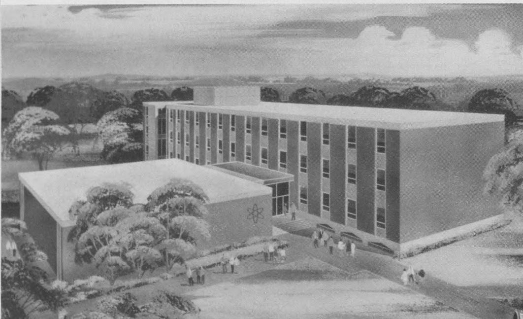
Construction has begun of new Science Building.
