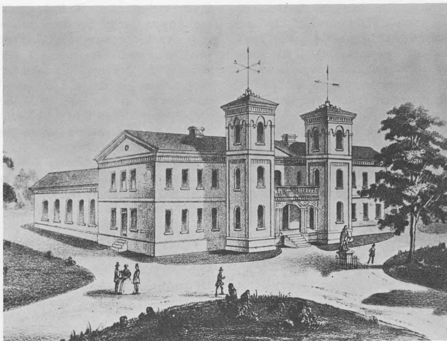
After fire of 1859, Richmond architect "modernized" building by removing third floor and dormer windows and adding Italian towers.
