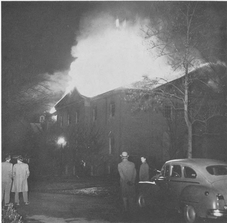
As volunteer firemen arrived "pent-up heat exploded in a brilliant fireball." Moments after this, roof collapsed.
