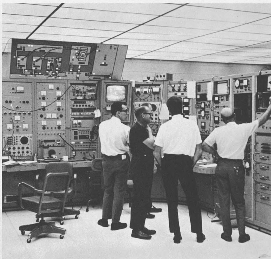
Scientists maintain watch over central control panel
