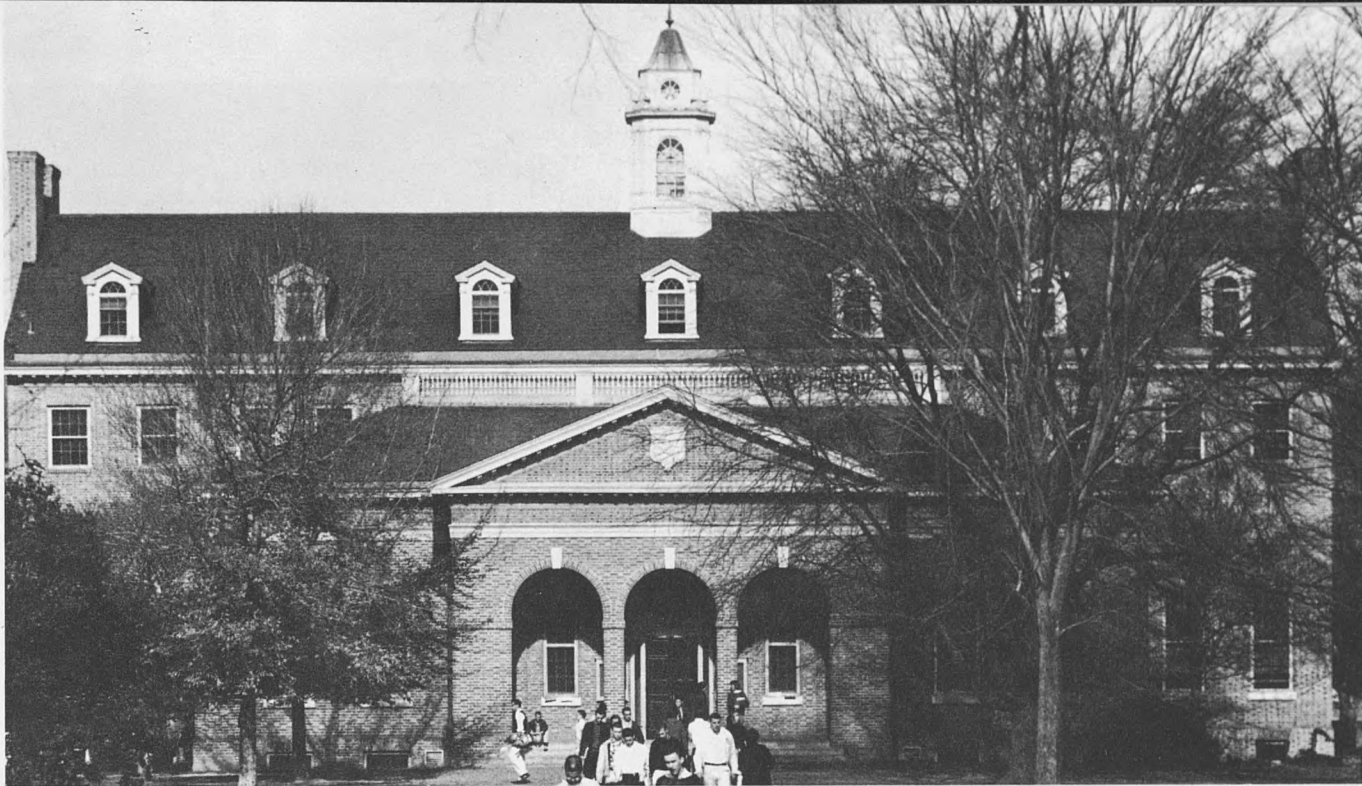
The Old Library was renovated for the Law School
