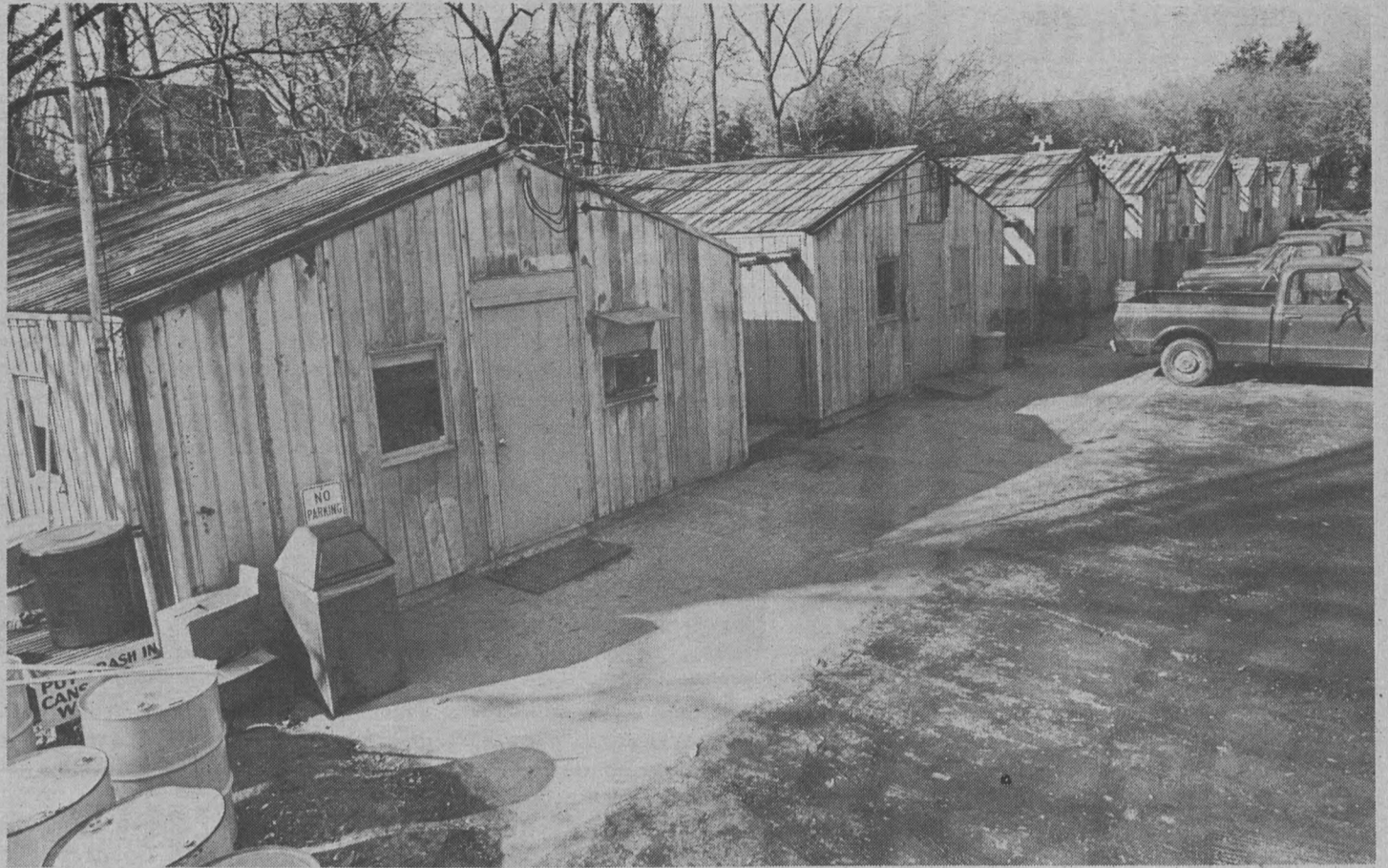
These are some of the buildings that would be replaced if William and Mary receives some $1 million in capital outlay money to renovate its plant services complex. The renovation is included in a list of capital outlay projects that would be funded by a $97 million tax package proposed by Governor Godwin. The package also includes money for a new law school building.
