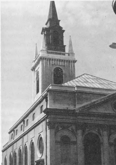
St. Lawrence Jewry, London (5), shown shortly after its restoration, whose steeple, like many of Wren's shorter spires, was built of wood covered in lead sheeting; St. James Garlickhithe, London (6), shown during post-war restoration that is now complete; Winslow Hall, Buckinghamshire (7), one of very few private houses definitely designed by Wren whose size and shape recalls some of the larger mansions built in Virginia half a century later; and Hampton Court Palace (8), a few miles up the Thames from London. Wren enlarged this Tudor palace, once the property of the notorious Cardinal Wolsey, and created a masterpiece in the Dutch taste for his stolid clients, King William and Queen Mary. (Photos by author)
