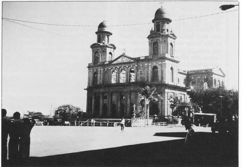
Cathedral in central plaza in downtown Managua. The roof and many of the interior walls were destroyed by the 1972 earthquake.
