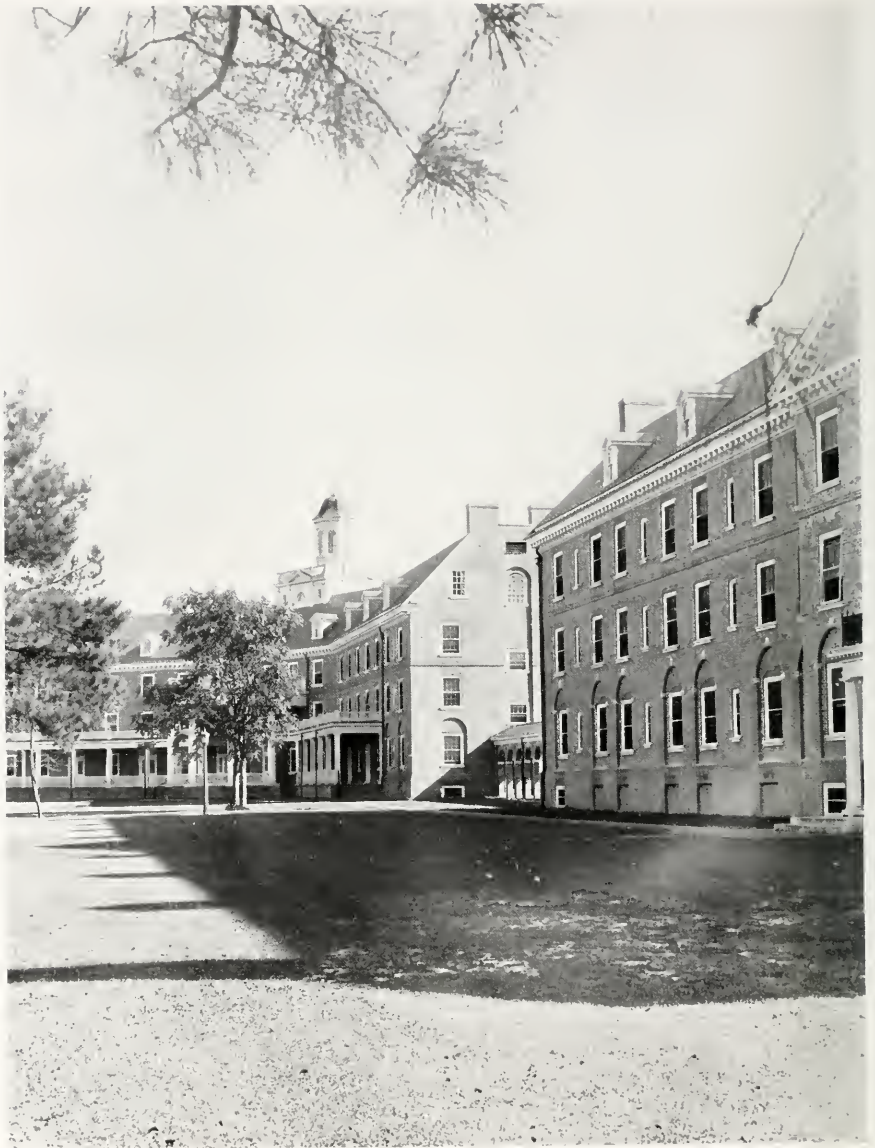
View of Chandler Hall and Barrett Hall
