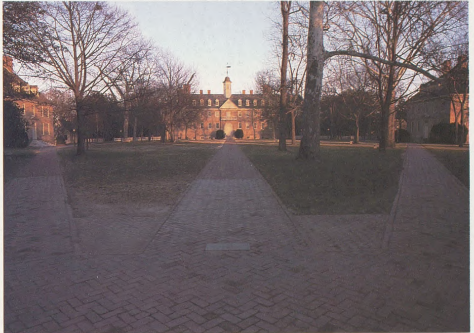
THE WREN BUILDING BY DAN DRY.
