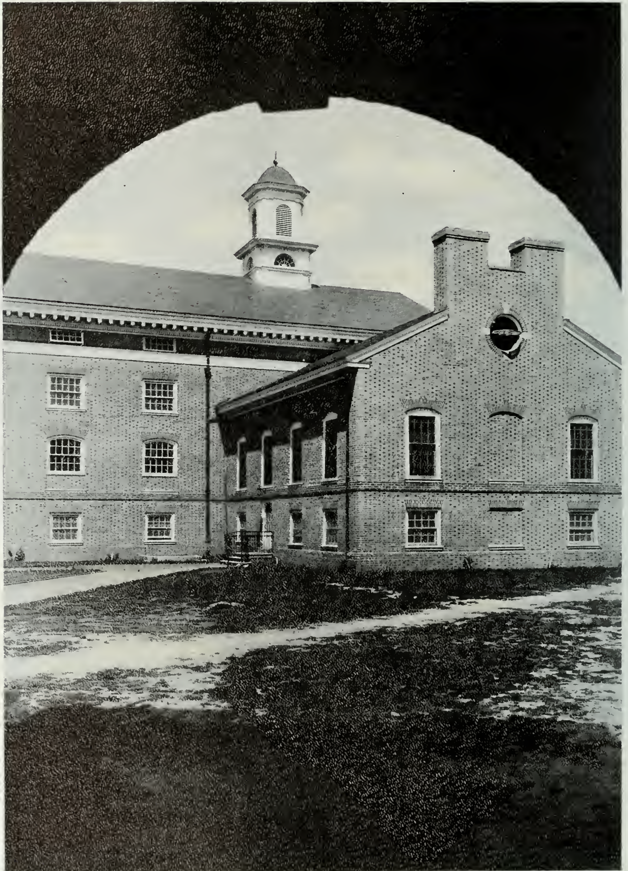
BLOW MEMORIAL GYMNASIUM
