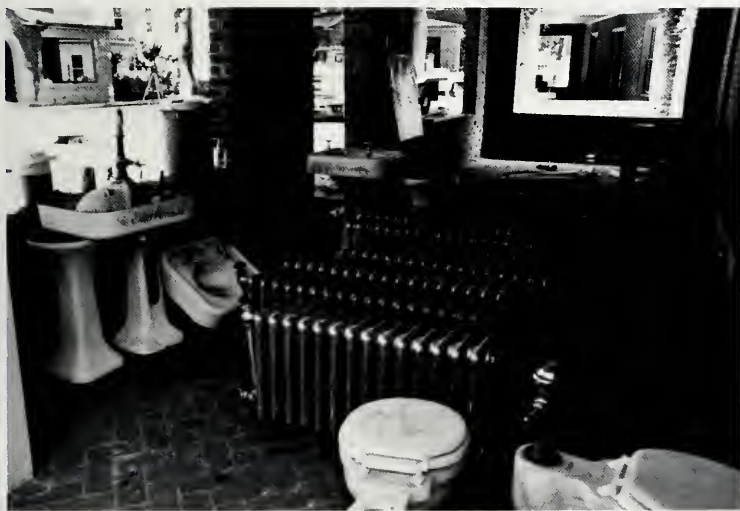
Misplaced plumbing litters the porch of Alpha Chi Omega during the ritual move to Randolph Residences because of sorority court renovations. — Photo by Chad Jacobsen.
