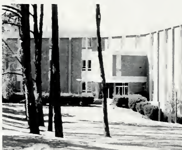
Housing a health hazard. Morton Hall is one of several academic buildings sprayed with asbestos. Some professors based in Millington and Morton refused to teach in the contaminated buildings. — Photo by Ben Wood
