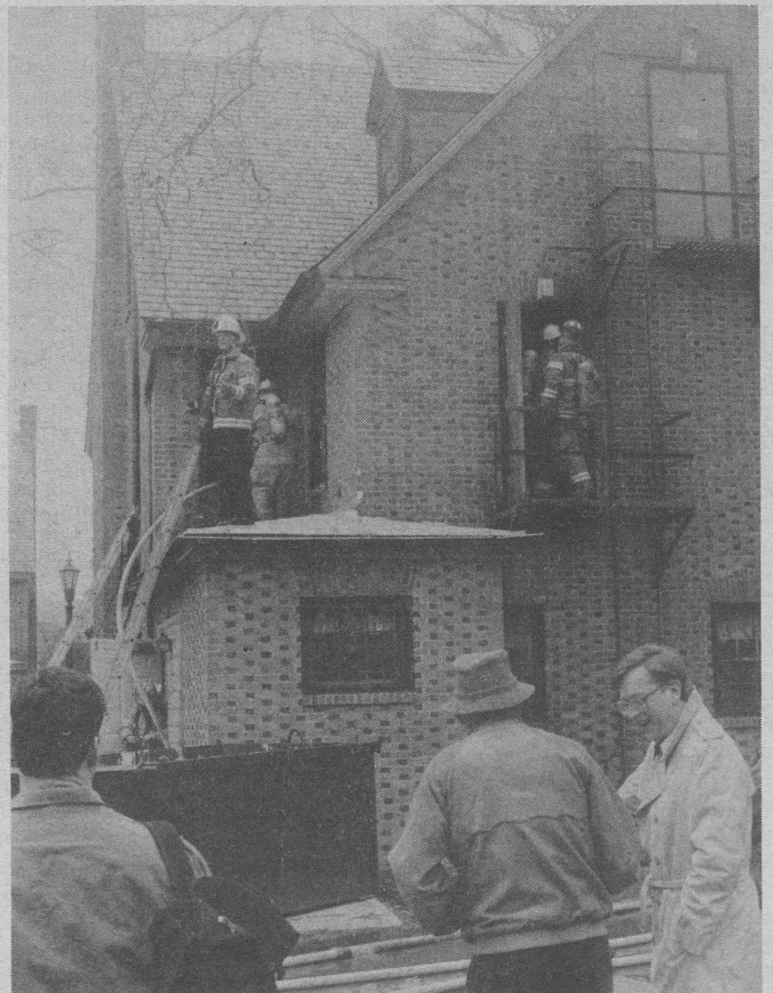
A fire that apparently started in a faulty appliance caused about $30,000 in the Chi Omega House over spring break. The blaze, which destroyed one bedroom and caused some water and smoke damage throughout the three-story building, was discovered by a student who went to the room to use a computer. Fire officials said the accidental discovery of the fire at an early stage enabled a quick response and probably saved the building. No one was injured.
