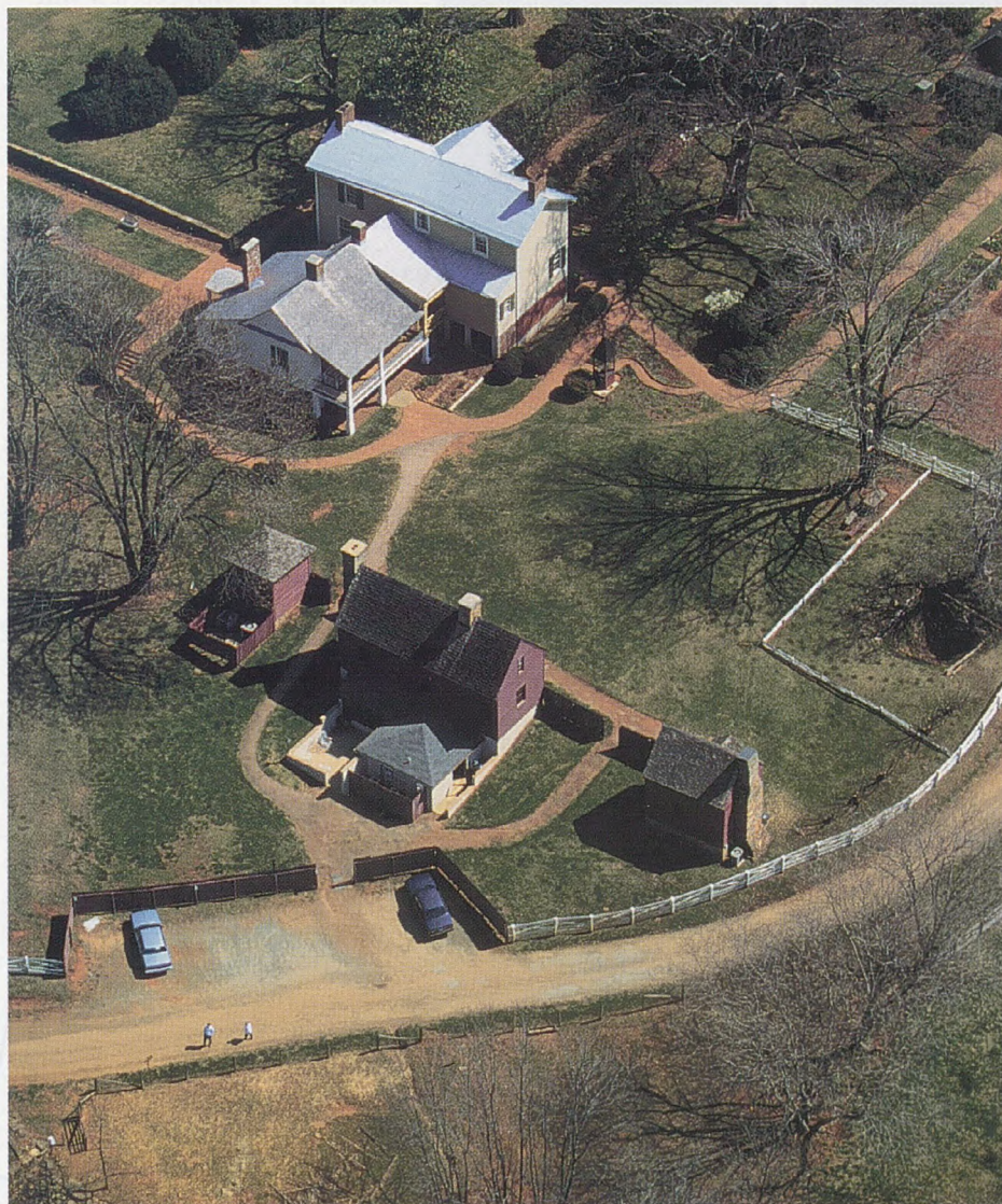
This view of Ash Lawn-Highland shows Monroe’s home (top) and the slave quarters (below).
