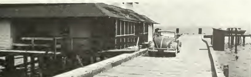
Dean William Hargis oversees a wide variety of facilities at Gloucester.
