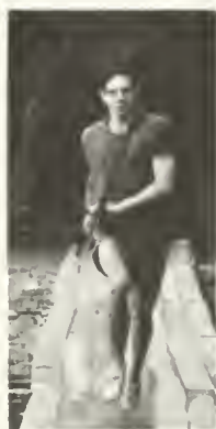
Start of vault.
