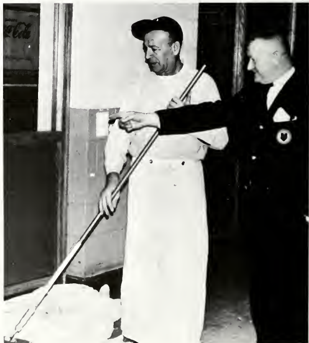
Colonel Warren Green superintends work in the Campus Center basement as the pool room becomes the "Sit 'n Bull" Room.
