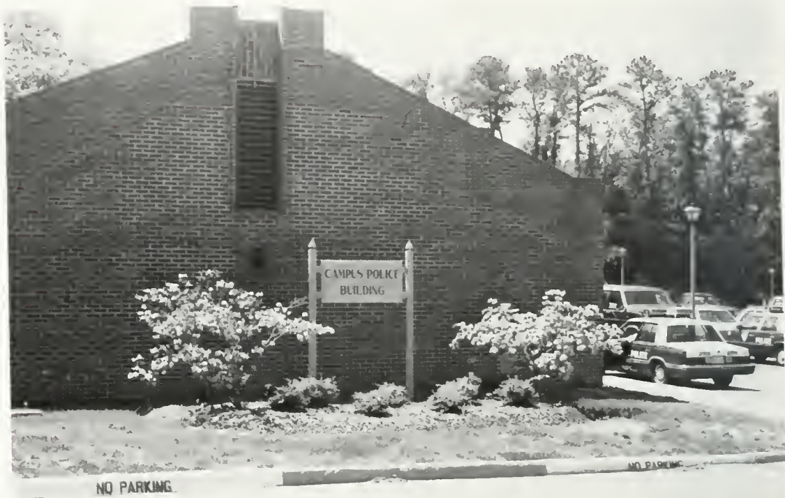
The campus police building as located behind the Campus Center and the mechanical building. The parking lot of the police station is the only parking lot found on the older side of campus, however, only faculty and staff are allowed to park there.
