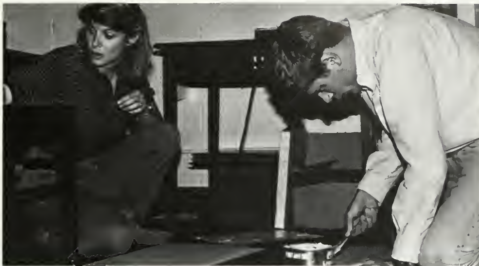
Right: Going beyond the call of duty, Business Manager Karin Magiera and boyfriend Rob Sedivy help in renovating the office by putting up new corkboard on the walls. This is Magiera's first year dealing with the yearbook and despite the fact she was responsible for money matters she often found herself doing layouts as well.
