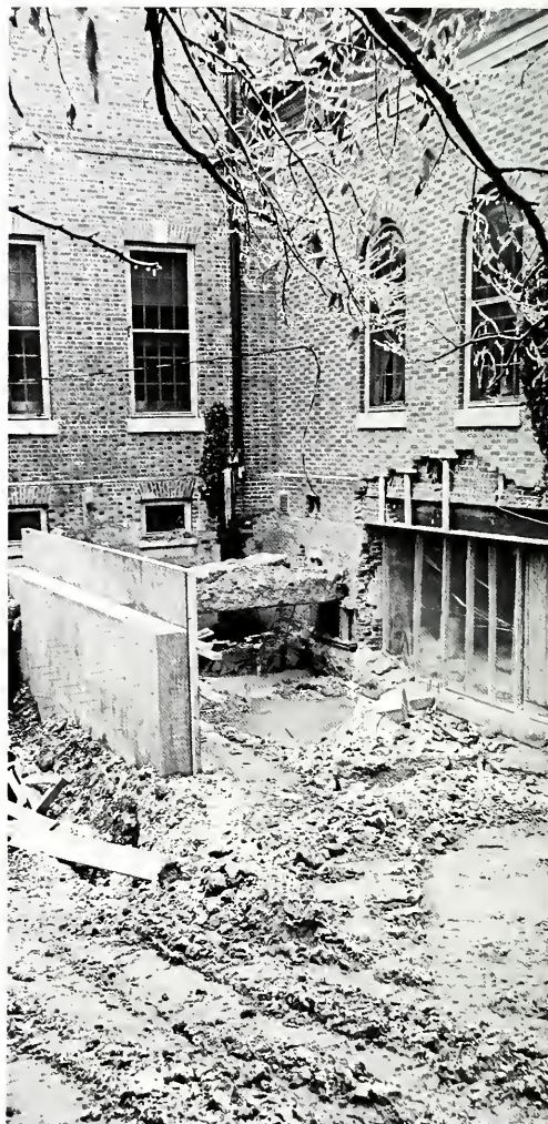
February's icy weather temporarily halted work on the Old Library.
