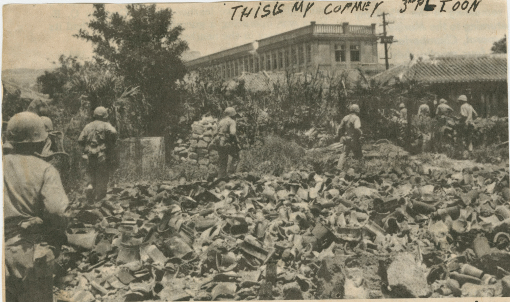
Few buildings remained standing amid the wreckage
