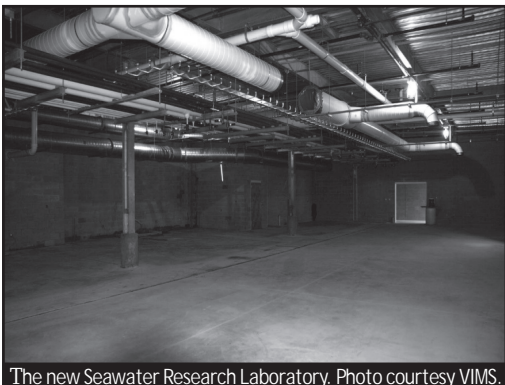
The new Seawater Research Laboratory. Photo courtesy VIMS.
