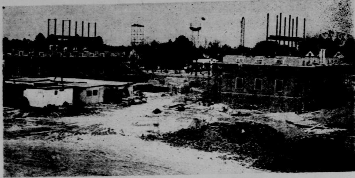
Construction continues on new men's dormitory.
