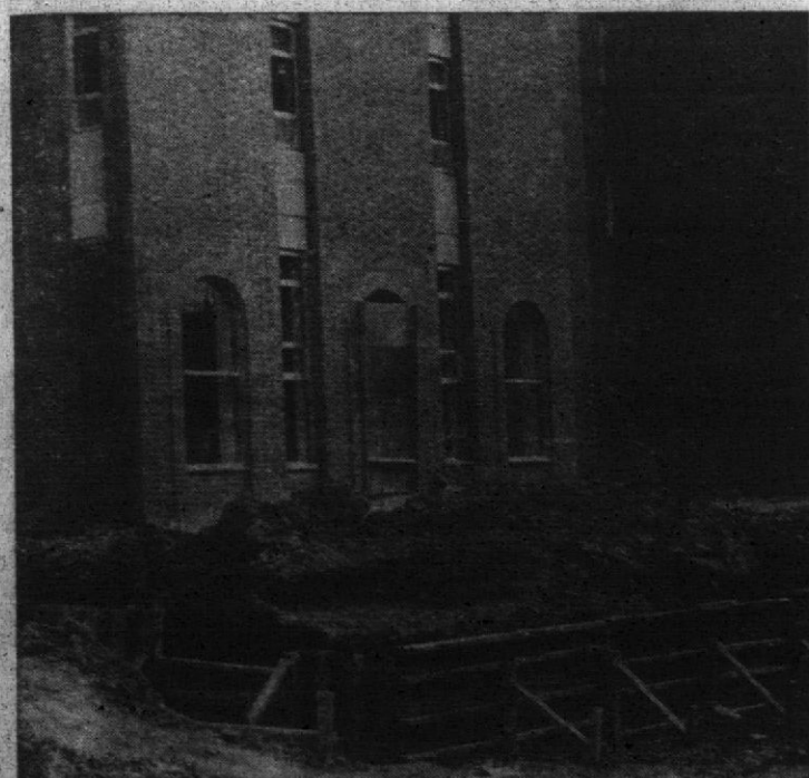
WORK'S NEAR COMPLETION
