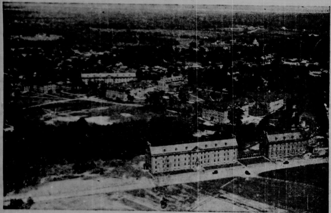
An air view of the College of William and Mary shows many of the new buildings. The women's dormitories are in the foreground. Other buildings seen include men's dormitories, the gymnasium, the science hall and the rich Beta Kappa Hall.
